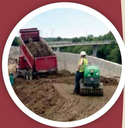
Construction of the first phase of the riverside promenade has begun.
